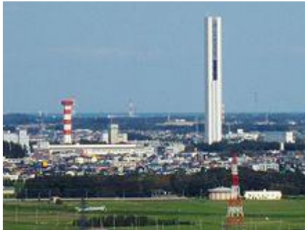
An elevator test tower
